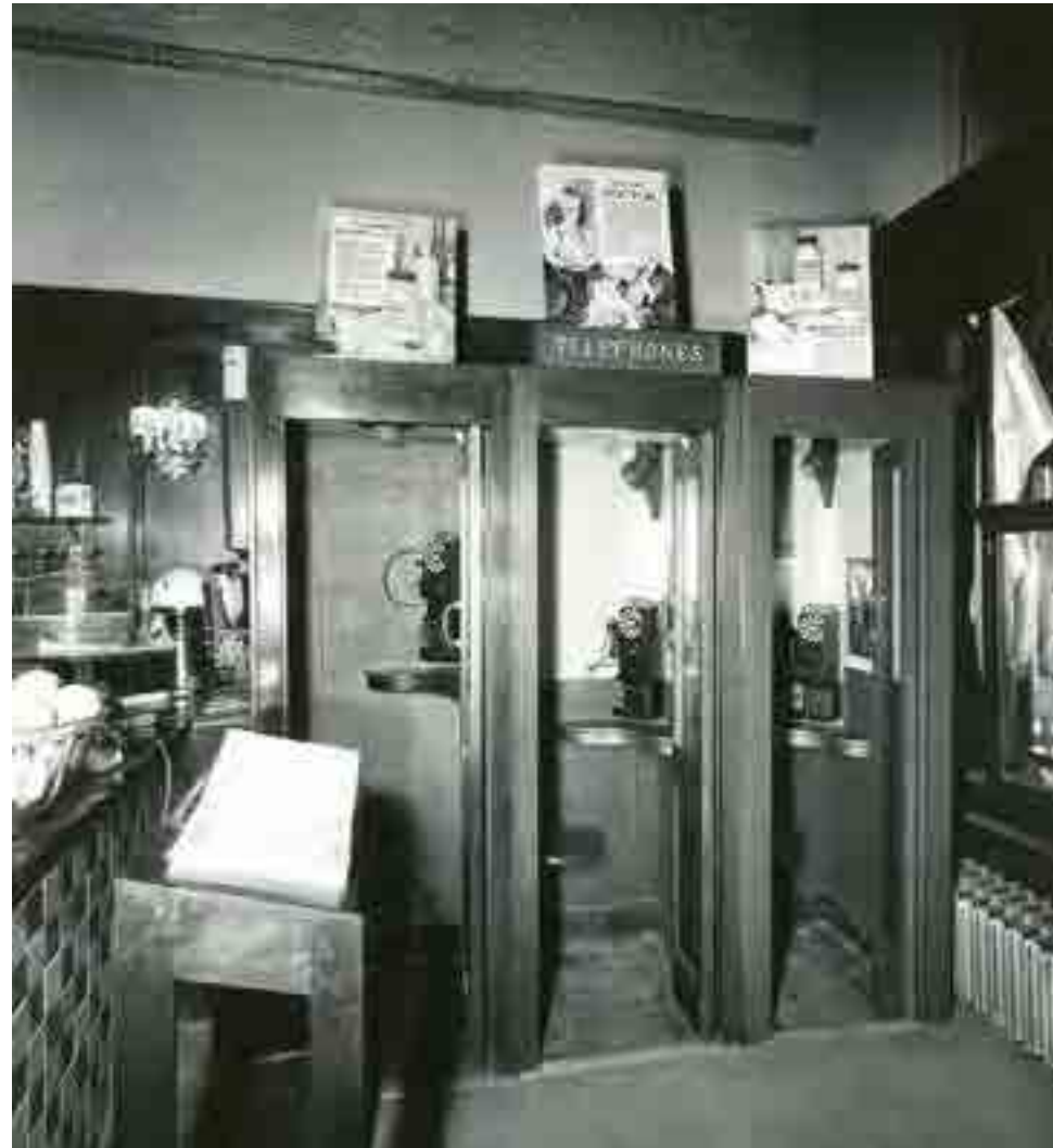
Indoor Telephone Booths in NYC (1940) Photo courtesy AT&T Archives and History Center
